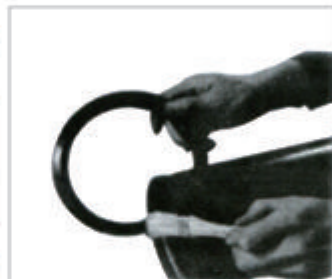
Lubricate gasket
