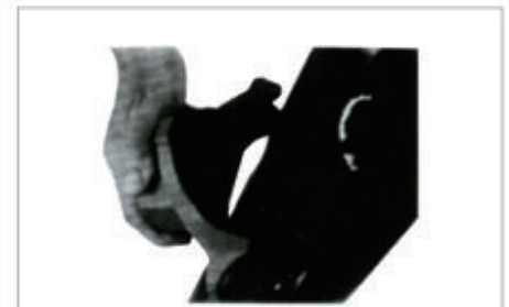
Gasket installation
