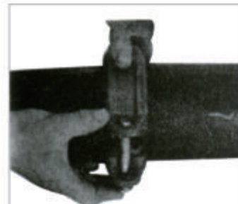
Housing installation
